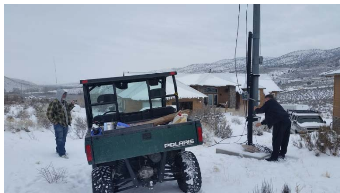
Mike Russo, N6EVG and Heiko Muench, KF7STT try their best for antenna repairs under challenging conditions. (Photo provided by Rick Crockett, WØPC)
