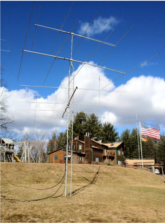
Another portion of the KC1XX 10 meter antenna system. These are dedicated to the second radio. (Photo - KM3T)
