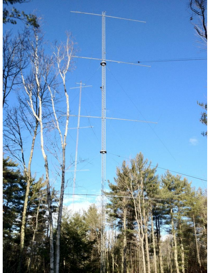
A portion of the KC1XX 10 meter antenna system. This is the 7/7/77 rotary stack. (Photo - KM3T)
