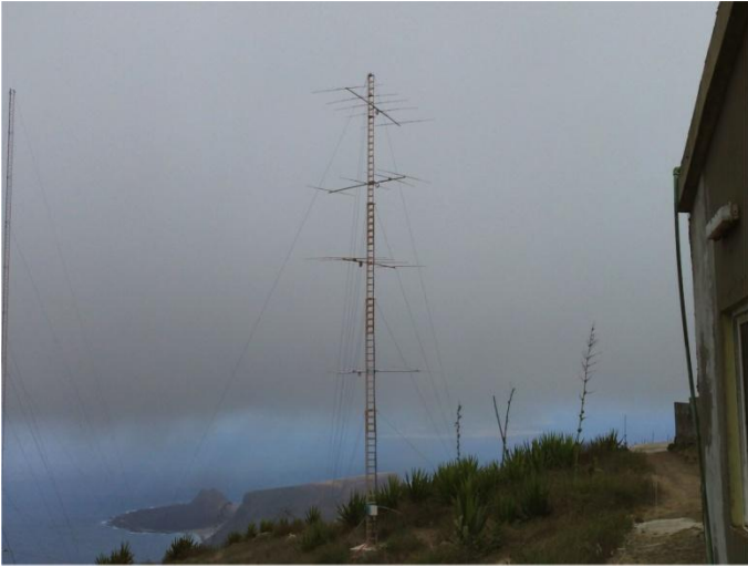
These are the 10 meter antennas at D4C. They can beam into any combinations of these antennas they want, up to and including all four for 360 degree coverage! (Photo - I4UFH)
