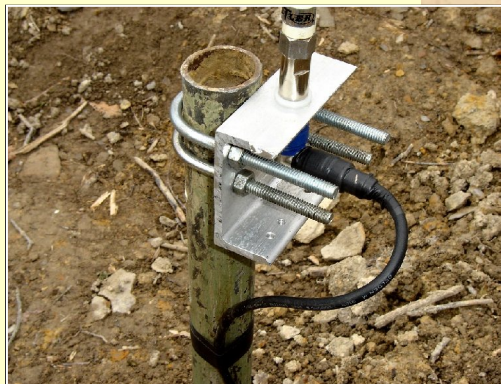
A piece of aluminum channel was used as the mount. Two U-bolts attached it to the pipe while the antenna mount is between them. There are various sources for the 3/8 by 24 thread antenna mount but Radio Shack was the closest.
