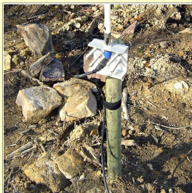
A 36 inch piece of 1 5/8 inch galvanized pipe is driven 18 inches into the ground. RG-8X coax is then taped to the pipe to provide strain relief at the PL-259 connector. Black electricians tape is used to weatherproof the connections.
